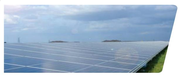
In addition, the half-cell technology powering these modules can also reduce both the internal losses between modules and the operating temperature in the case of actually running the power station, thus supporting steady operation and lowering future maintaining costs.
